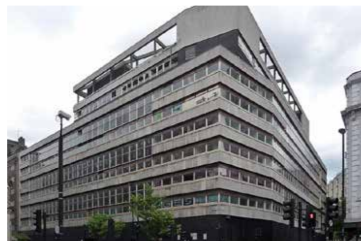
The Post Building was vacant for a number of years before its recent redevelopment for office space.
