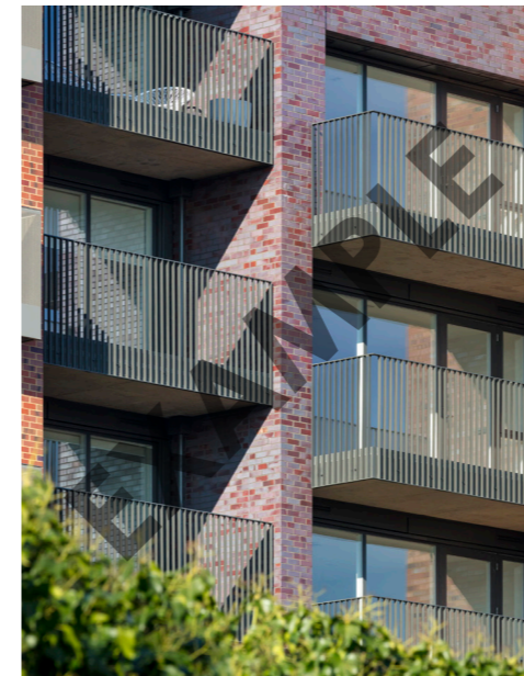
Spacious balcony connected to bedroom - EXAMPLE
