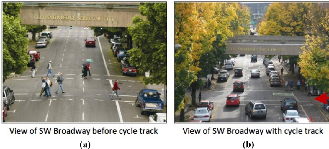
1 2 3 FIGURE 1 Cross-sectional configuration of SW Broadway (a) Prior to cycle track 4 and (b) with cycle track implementation
