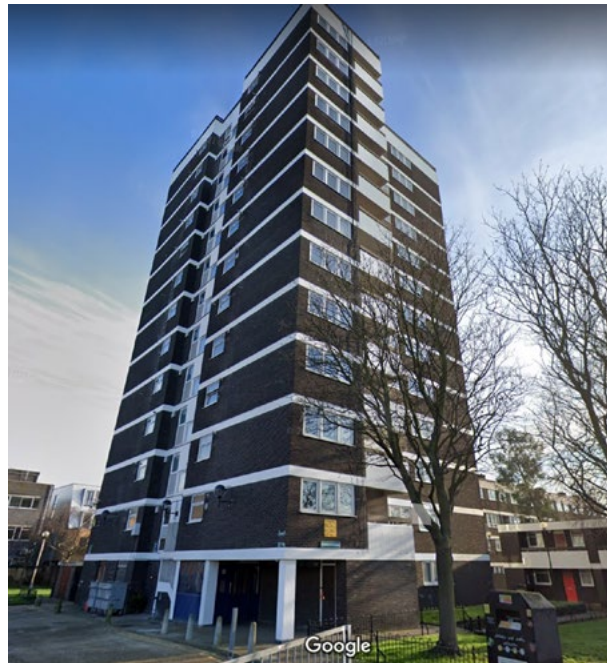
Image 2.4: Point block building (credit: Google)
