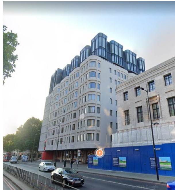
Image 2.9: Hotel building (The Standard Hotel) (credit: Google)
