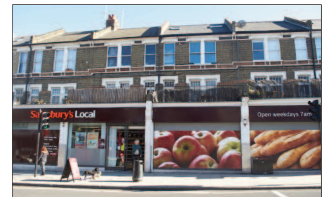
▲ Sainsbury's Local 126-132 Fortess Road
