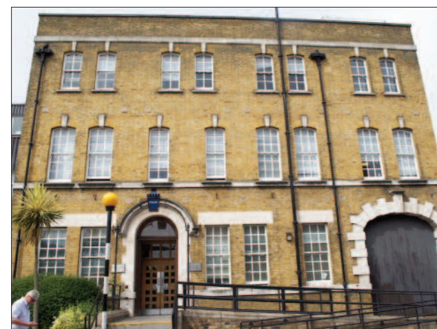
▲ The Police Station, Holmes Road. Grade II listed
