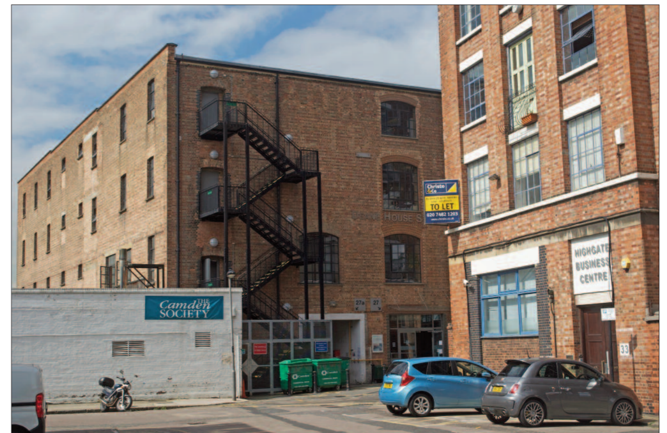
▲ Part of Highgate Road Section
