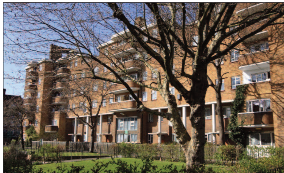
▼ Willingham Close Estate, NW5 2UY, is composed of three blocks. Willingham was built first as mews properties and took a direct hit from a bomb. It was rebuilt, followed by Rosemary and Margaret House. The Estate was designed and built by a St Pancras in-house team. It was opened in 1952. Cecil Rhodes House in Camden Town was built using the same basic design. One of the residents says, "The Estate is a wonderful example of council-built buildings. The layout, either by design or luck, has produced a great community spirit among us all and I am a great believer that buildings do affect how people live."
